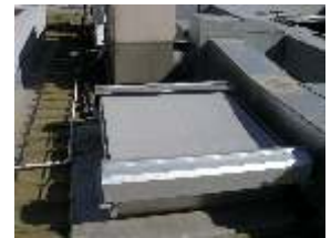
horizontal fixed guide awning over skylight
